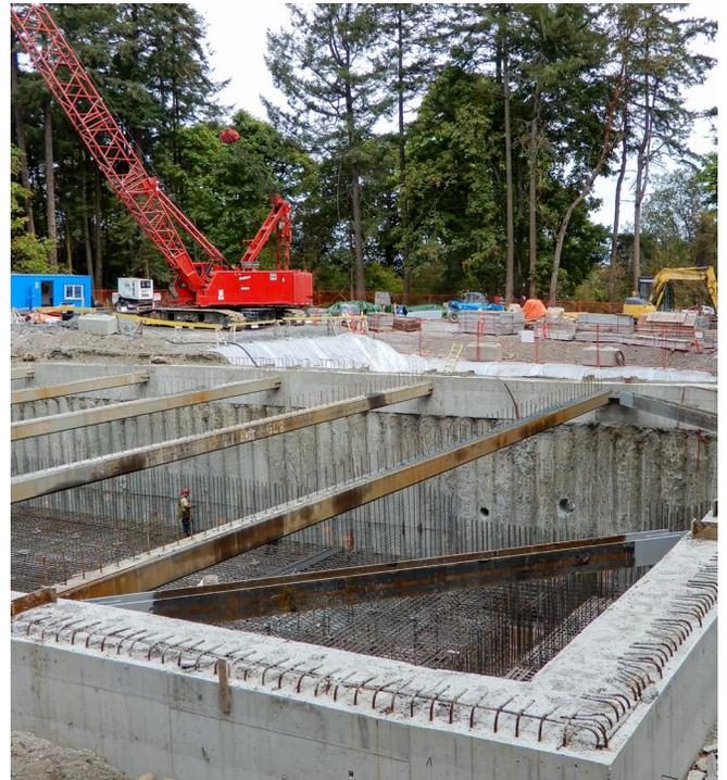
The concrete used for the secant piles contained Xypex Admix C-500 to permanently protect the reinforced concrete and minimize water infiltration during excavation and construction of the tank. Xypex Admix chemical treatment reacts with cement and the byproducts of cement hydration to fill the capillaries in the internal structure of the concrete, creating a non-soluble crystalline matrix. The result is concrete that prevents water penetration for its entire service life.
